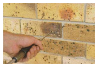
Inserting Tie into wall
