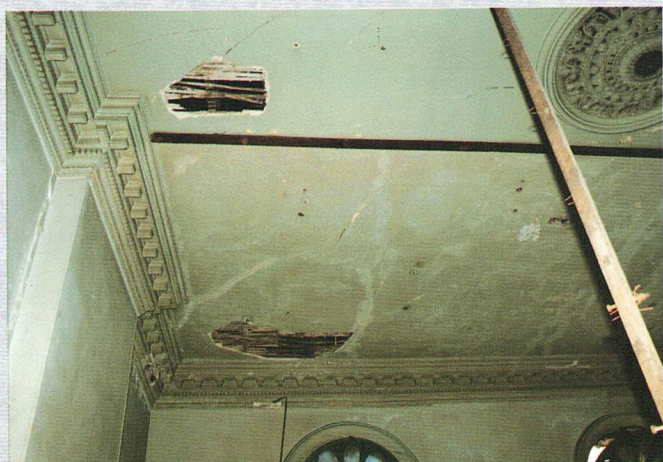
Ornamental lath and plaster ceiling requiring reinstatement
