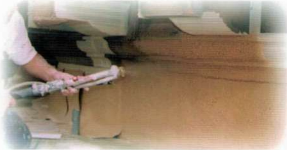
Spray Application of Cocoon
