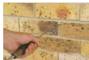
Inserting Tie into wall
