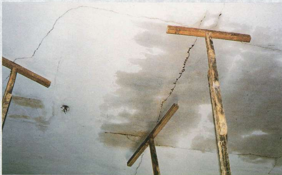
Penetration of adhesive and main propping areas
