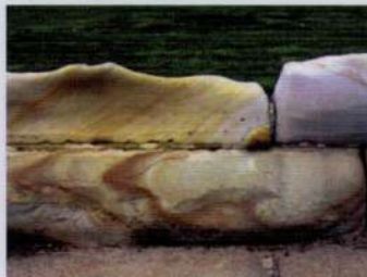
Salt Affected Masonry
