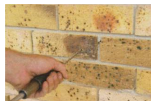
Inserting Tie into wall
