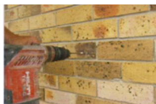
Drill Pilot Hole
